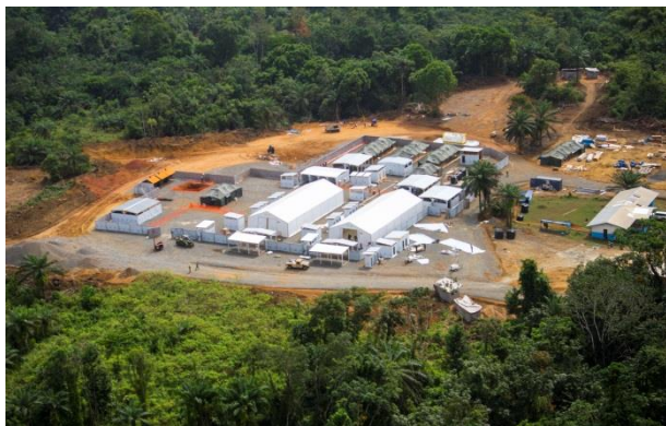
An aerial photo of the Gbediah Ebola treatment unit, the last scheduled ETU to be built by JFC-UA, 22 December, 2014. US Army photo, JFC-UA Public Affairs/Released
