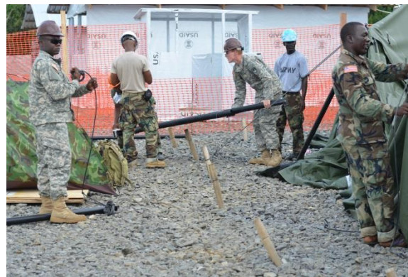
Soldiers of the 62nd Battalion, 36th Engineer Brigade, from Fort Hood, Texas and the Armed Forces of Liberia work together to complete the Sinje ETU, 19 November 2014. US Army photo/Released
