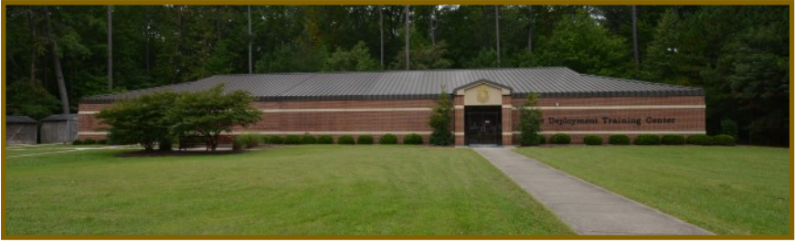
JDTC Resident Training Facility, Fort Eustis VA
